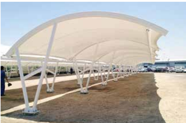
Car Parking Sheds
