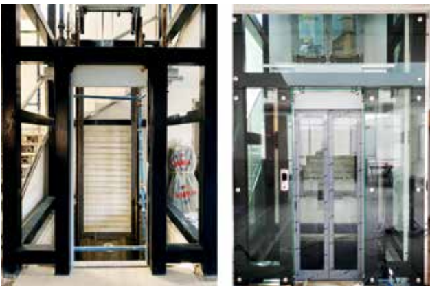
Lift Frame with Cladding
