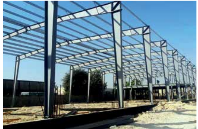
PEB Steel Framing
